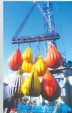
Load test with water weight bags 250 tons
